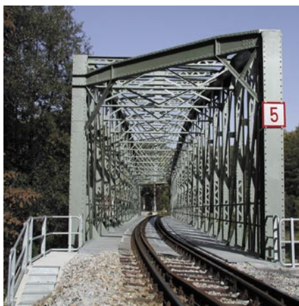
Railway bridge in the Kamptal/Austria
